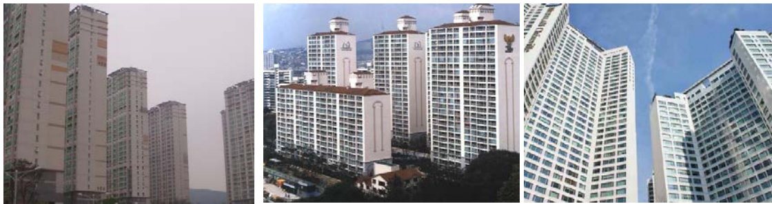
Fig. 1. Typical Korean apartment buildings.
